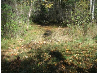
This is the driveway embankment blocking east channel from Little Round Lake off Thunderbird Road.
