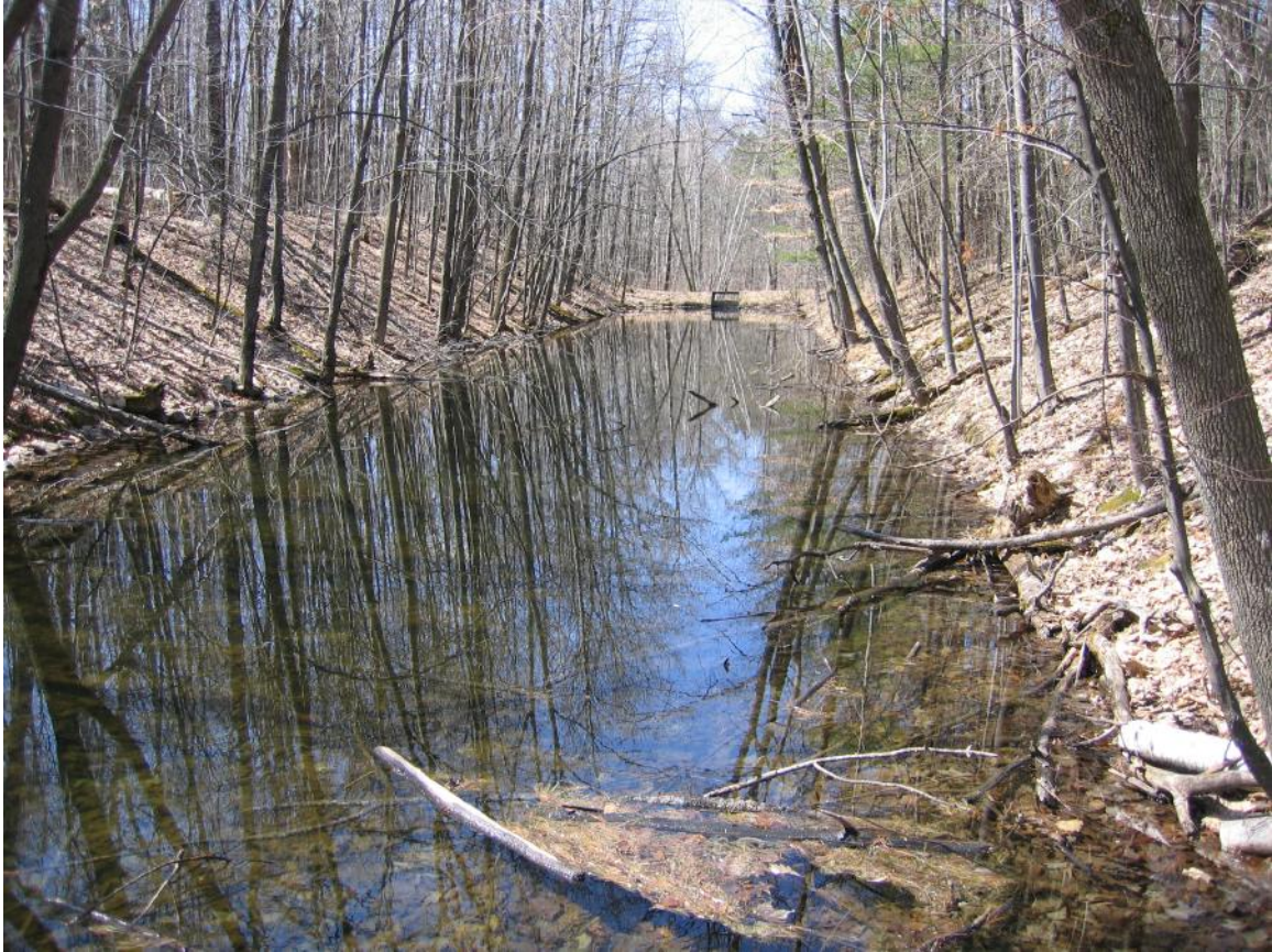
The Diversion canal upstream of dam.
