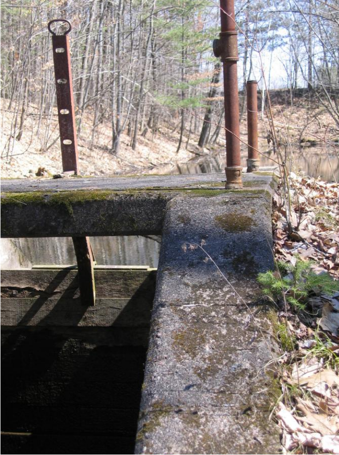
Looking at dam and pool upstream of dam.
